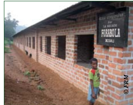
Photo 2.3: School constructed by a logging company
